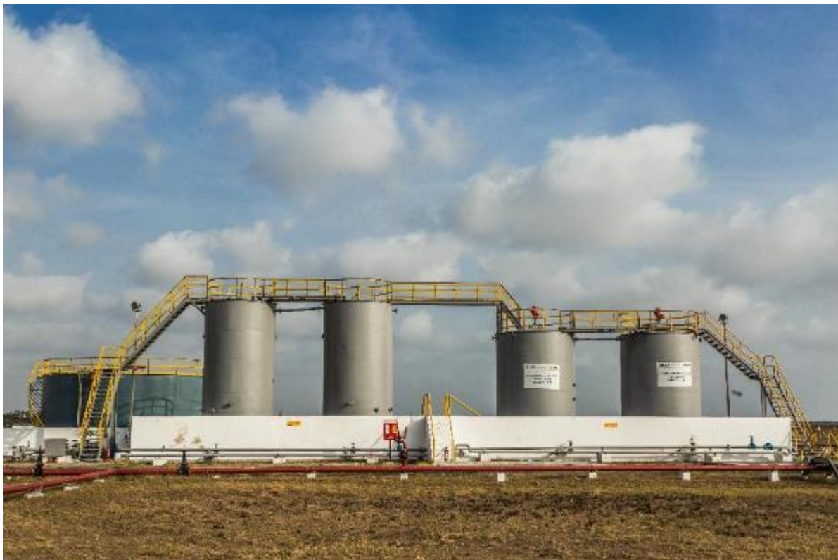
Figure 4: Bhandut Production Facility
