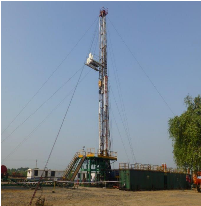
Workover rig on location
