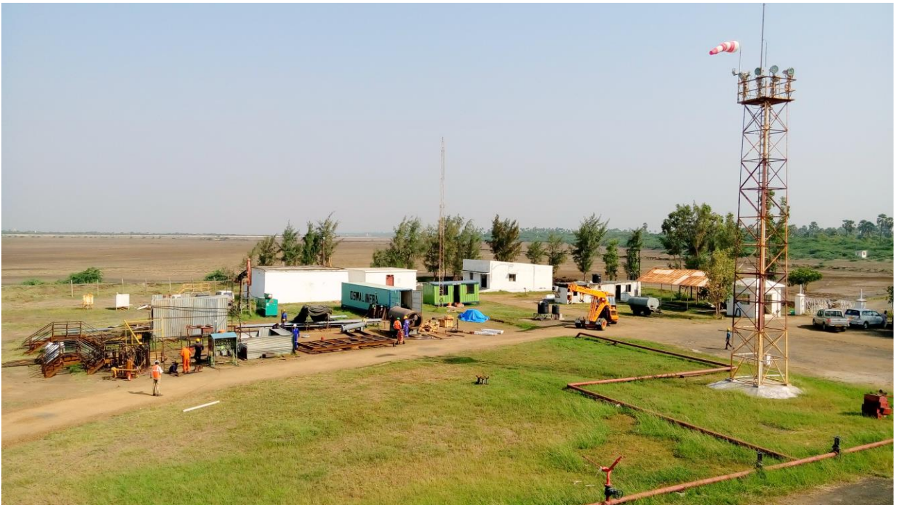
Bhandut Field during construction
