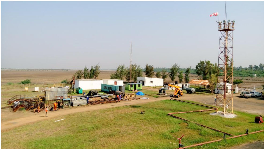
Bhandut Construction activities
