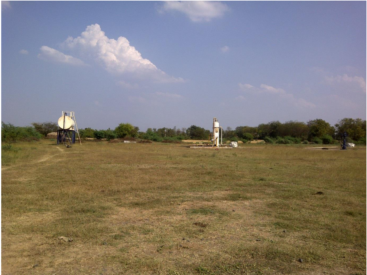
Cambay-73: Before commencement of construction activities
